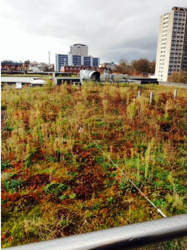
Image 4: view looking West at roof level of Worcester Point
